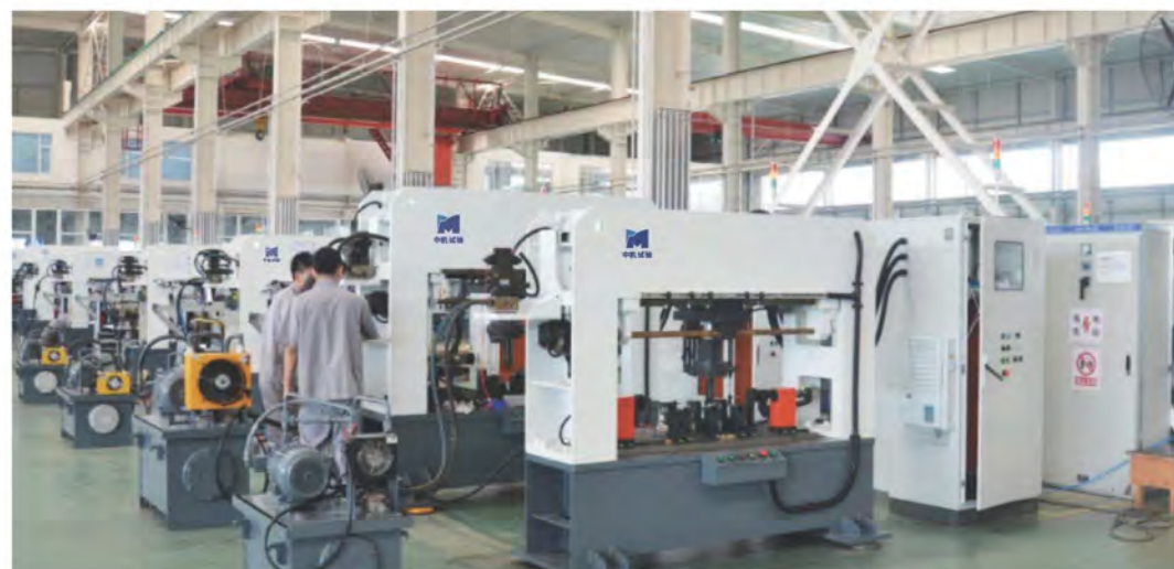
03 调试现场 Commissioning site
